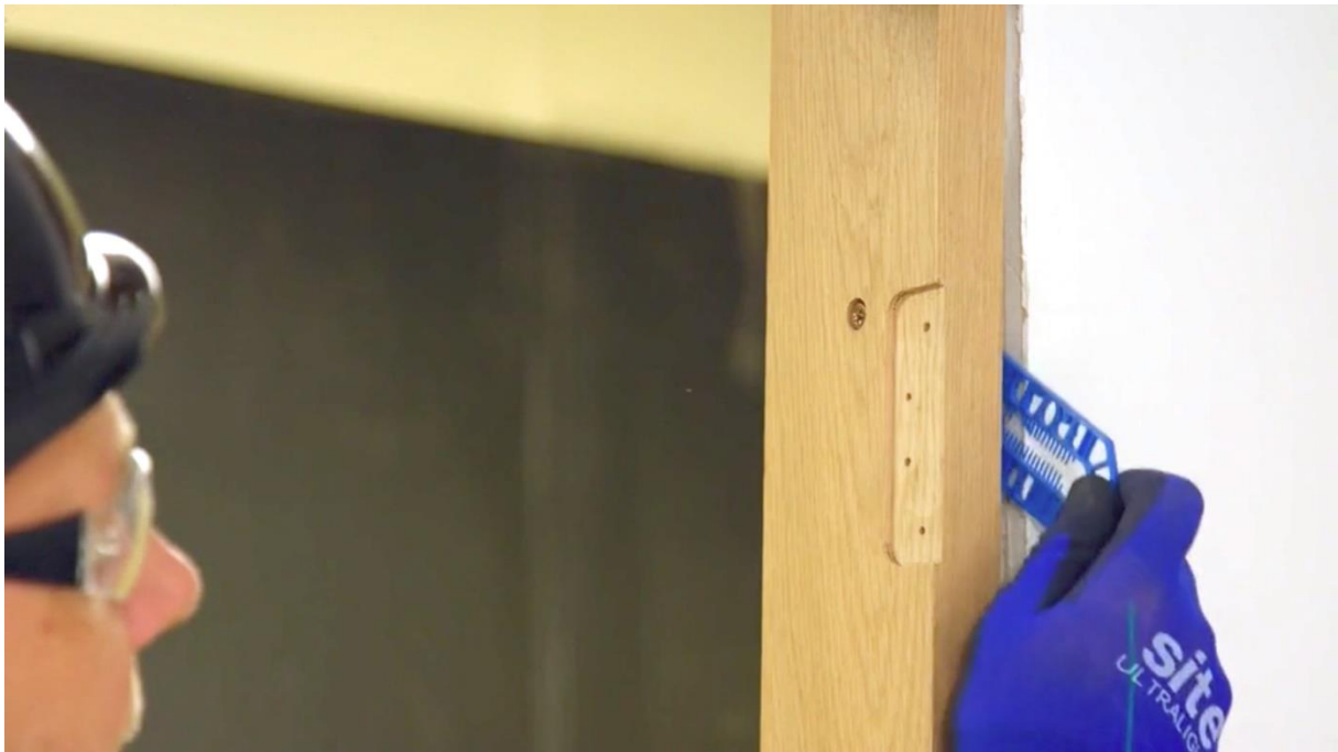
Figure 5: Generic example to Install packer
