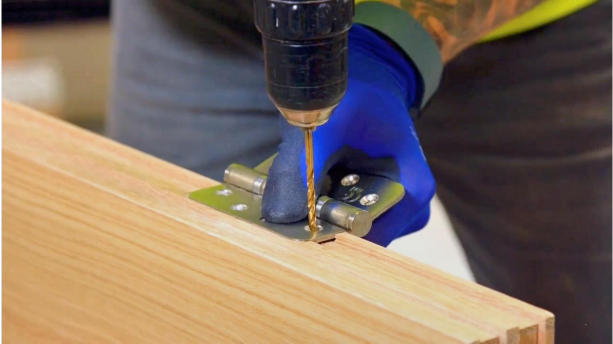
Figure 4: Generic example of fitting the hinges
